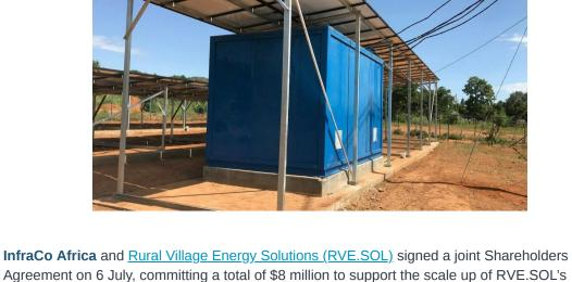
To date, RVE.SOL has established 20 operational mini-grids in the country. With support from InfraCo Africa, the project will build an additional 22 mini-grids across Busia County, in northwest Kenya. Incorporating battery back-up, the mini-grids will range in size from 10 – 60kWp, totalling 512kWp. A modular design enables the company to respond to changing electricity demand over time. The project will empower over 7,000 new rural electricity connections through a mix of
